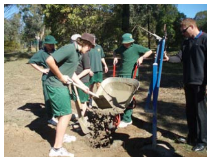
Students cementing the corner posts
